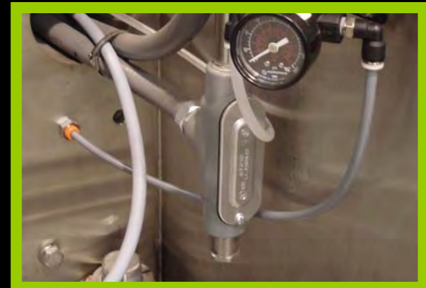
Drip Drains for all Junction Boxes and Low Wiring Points
